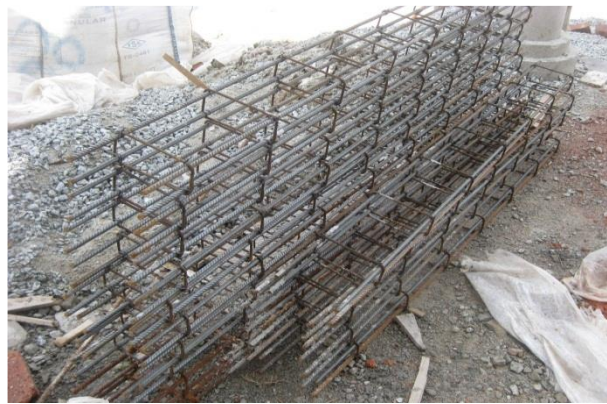
Besi tetulang (reinforcement bar)
