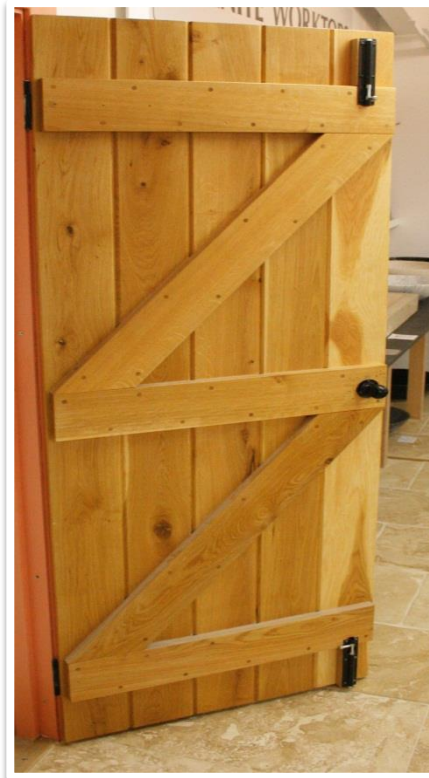
Beroti Dan Berembat (Ledged and braced)
